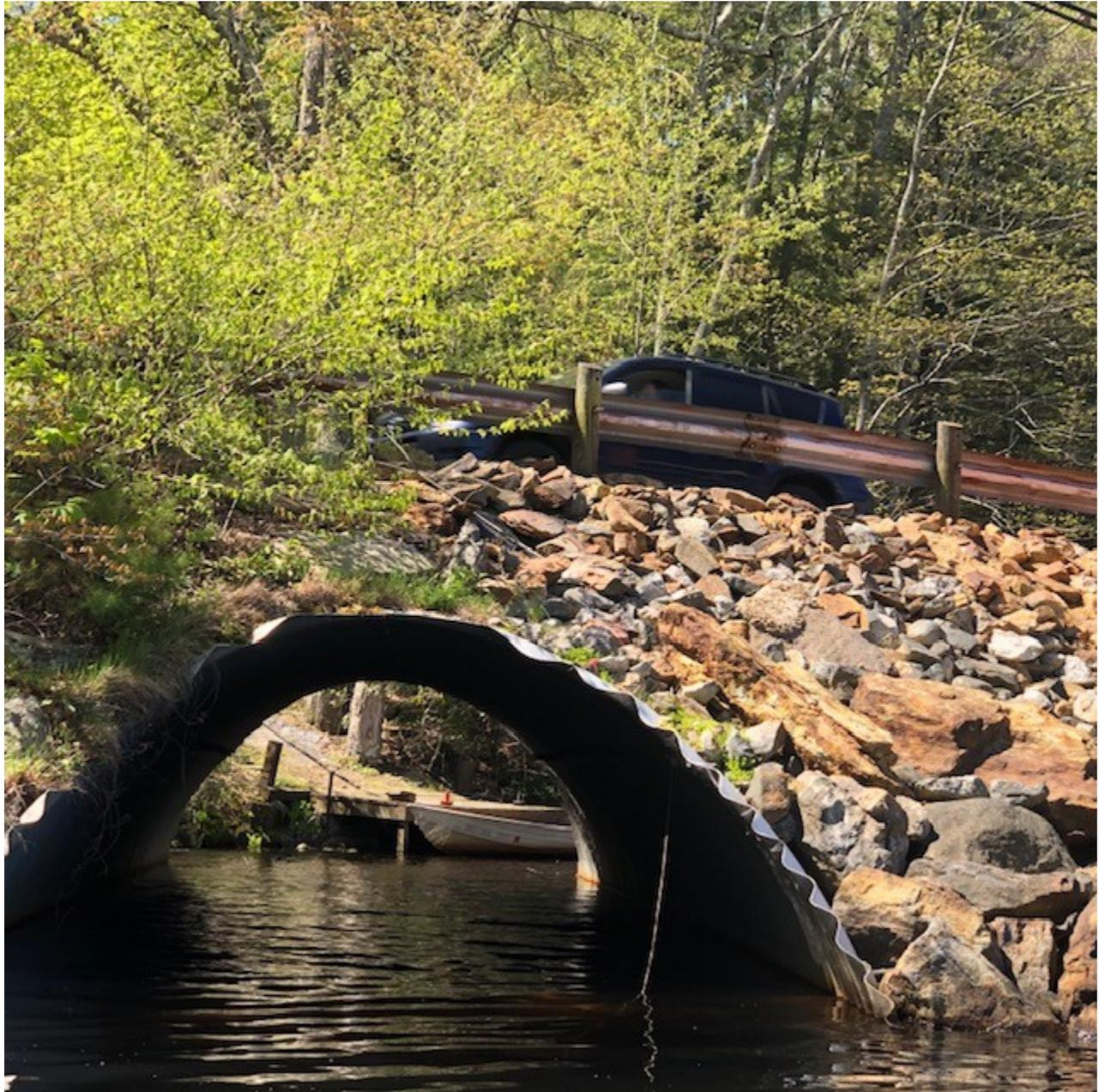
However, since the causeway dammed the water up to five foot and six inches above normal water-level, the culvert was submerged and was unable to carry the water of Browns Brook, the water found
