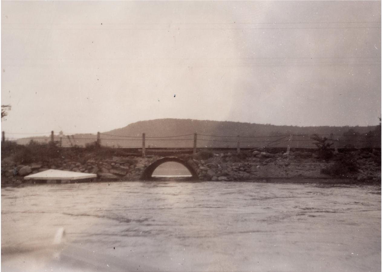
This culvert, which was unable to handle the water of the 1955 flood, seems to be larger than the one put in place during reconstruction of the causeway after the flood of 1955.
